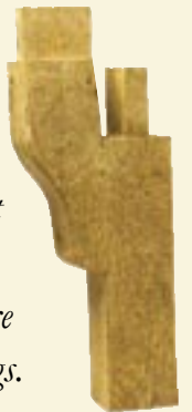
A Jowl, the enlarged head of a main post
