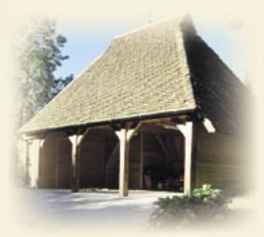
A Jowl, the enlarged head of a main post
